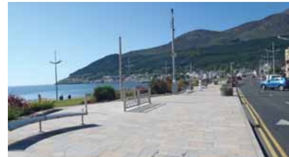
Public Realm: The Newcastle Public Realm scheme was implemented in 2008 and has completely rejuvenated the town centre and promenade. Footfall has subsequently increased dramatically.
