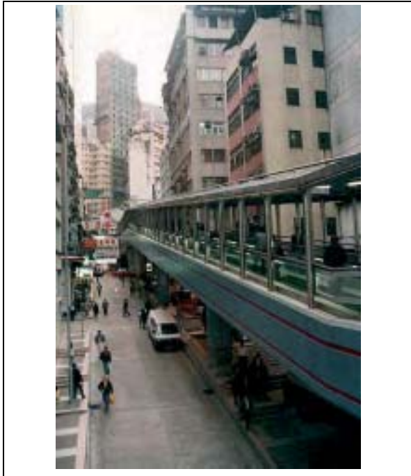
Figure 7.2 Outdoor Travellator (Hong Kong)
