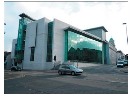
The remodelled Town Hall viewed from the south
