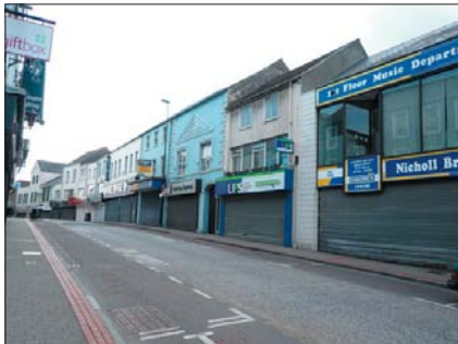
Poor quality shopfront design exacerbated by roller shutters
