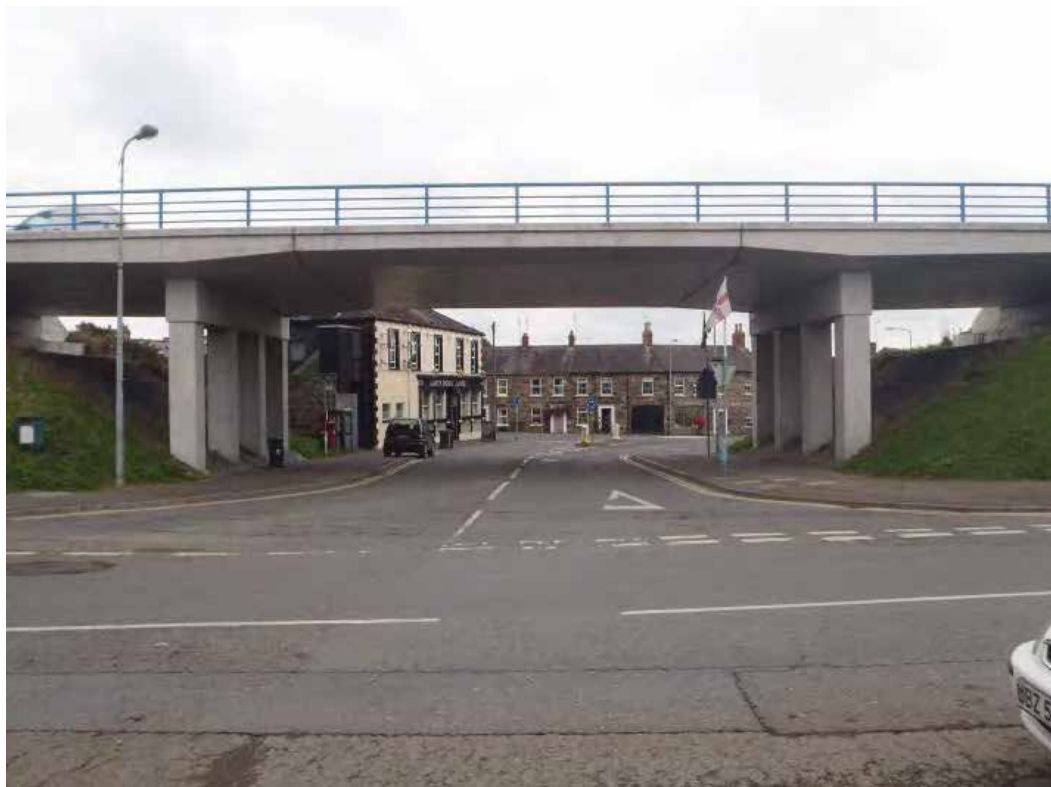
Figure 9 - By-pass infrastructure creates a physical barrier
