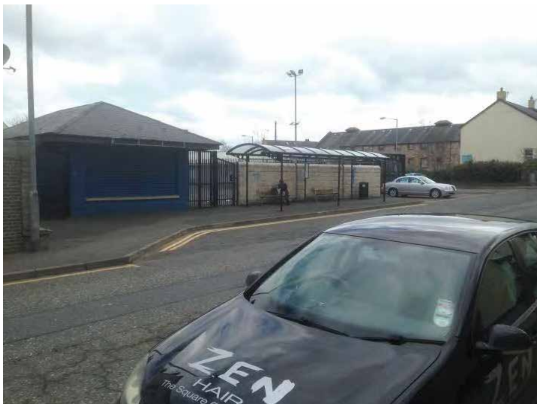
Figure 15 – Low quality bus shelter environment
