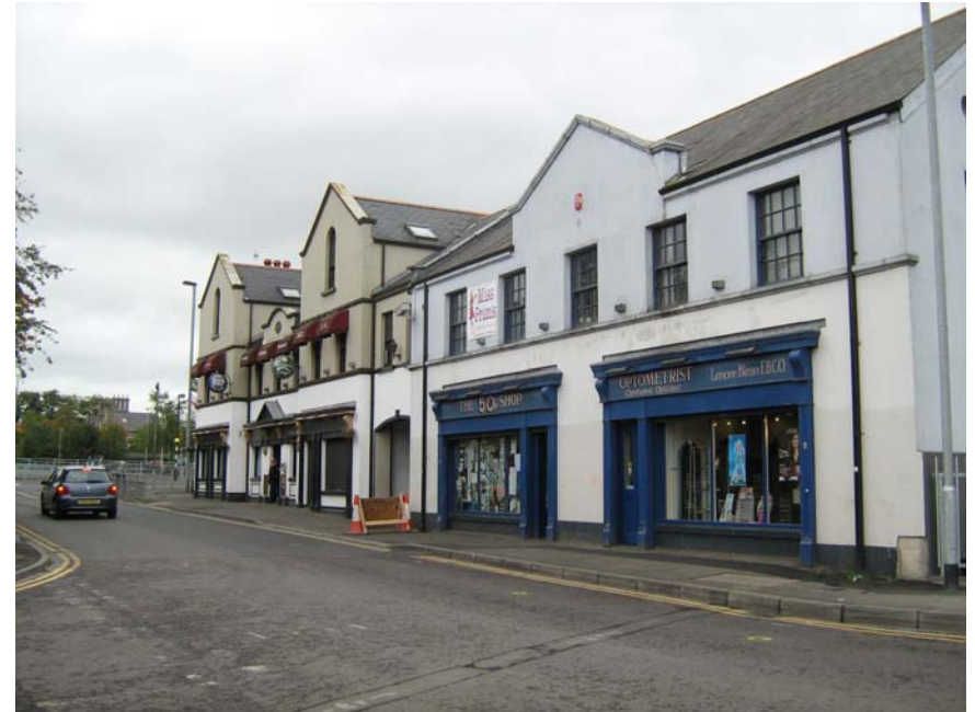
Photo 9: Railway Street (Site 3b)
