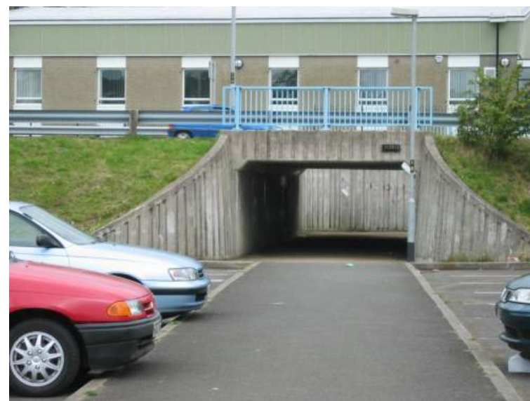
Photo 1: Subway under Castle Way from Central Car Park
