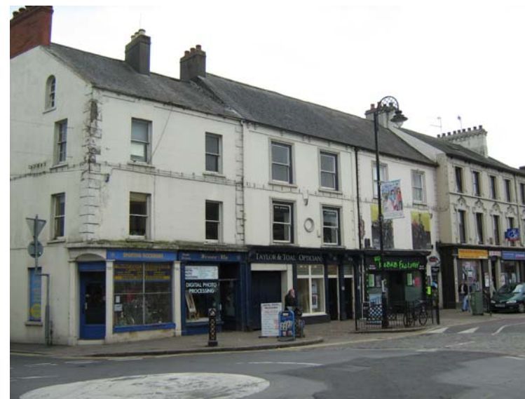
Photo 15: Poor quality building frontages on High Street
