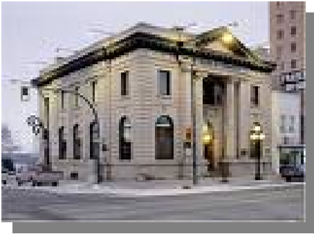
Bank Services Building
