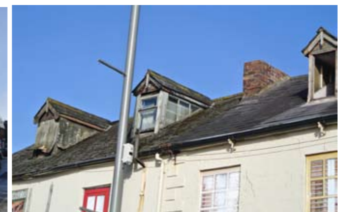
Vinyl insertions on Perry Street, with reference to 'glazed cheek' dormers still present.
