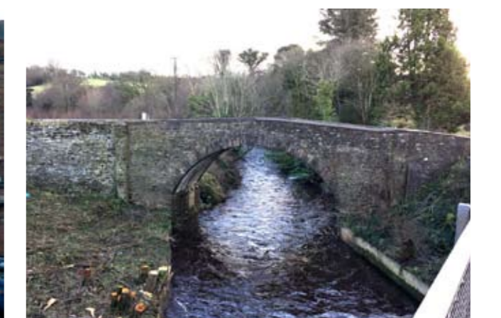
(above) Burntollet Bridge before its demolition.
