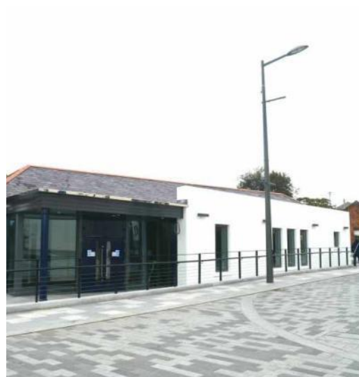
The unlisted former stable block with internal heritage features preserved.
