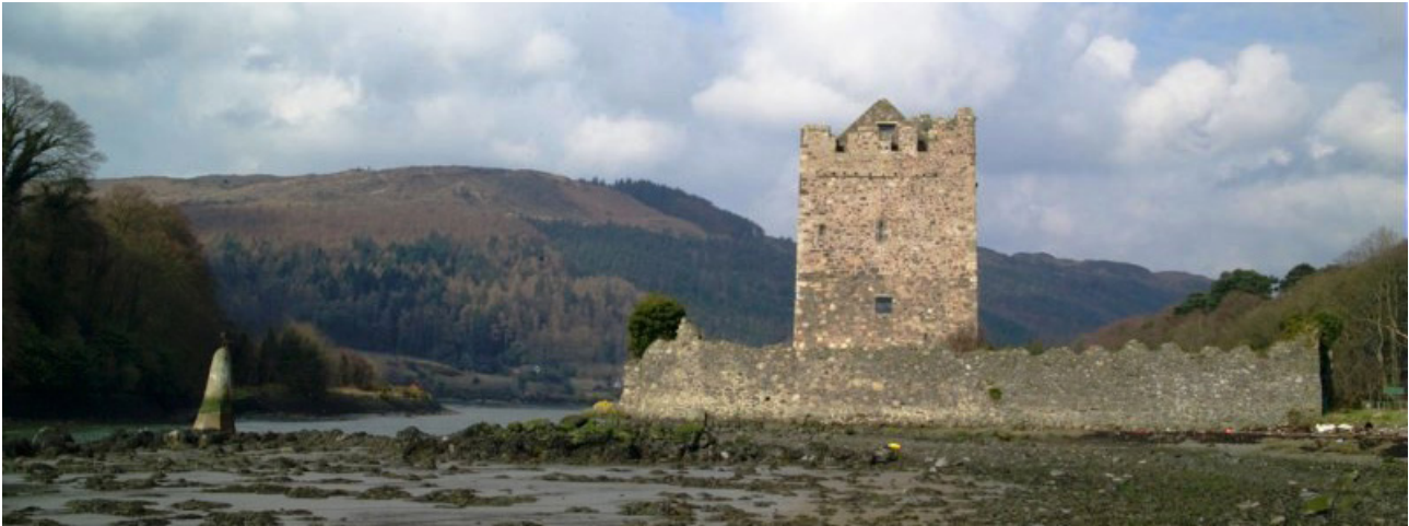
Narrow Water Castle, Co. Down. This 16th-century castle sits at a crossing point on the Newry River close to where it enters Carlingford Lough. The well-known tourist views of the site are an important aspect of the castle's setting and cultural significance.
