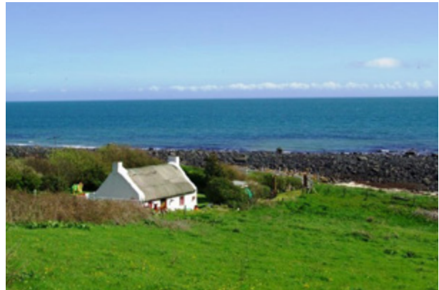
Cloghfin, Islandmagee, Co. Antrim. A listed thatched cottage which sits comfortably within a rural coastal setting.
