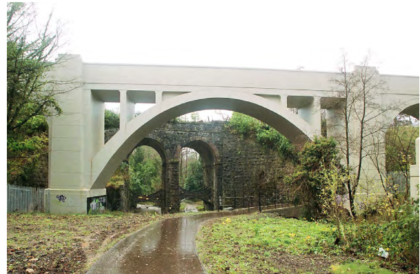
Railway Viaduct, Newtownabbey (HB21/10/001B - Grade A)
