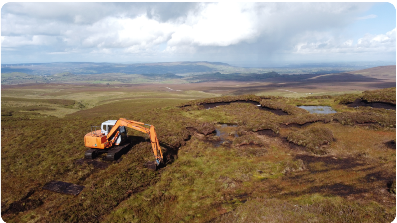
Digger installing peat dams, Cuilcagh, Co. Fermanagh, © Ulster Wildlife Trust.
