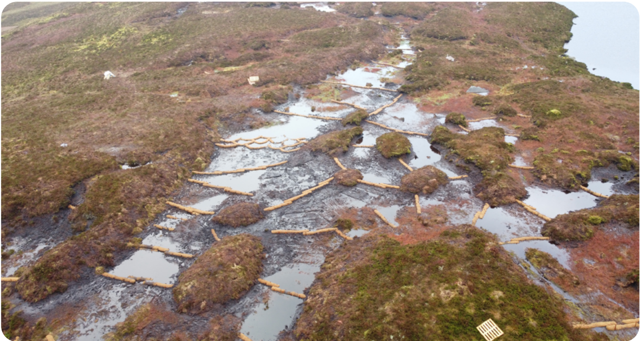
Use of coir logs for peatland restoration © Ulster Wildlife Trust. Coir logs can be used in areas to reduce impact.
