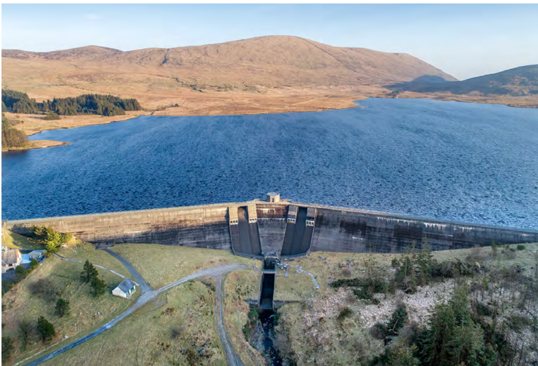
Spelga Dam, Ballynanny and Stang, Co. Down DOW 048:500. View of the dam with triple syphons and octagonal tower at the centre. Proposed to HMC as a scheduled historic monument (HM560).
