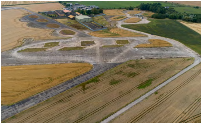
Cold War Readiness Platforms, Ballykelly, Co. Londonderry DHR 00029:50, 51, 52, 53. Proposed to HMC as a scheduled historic monument (HM548)
