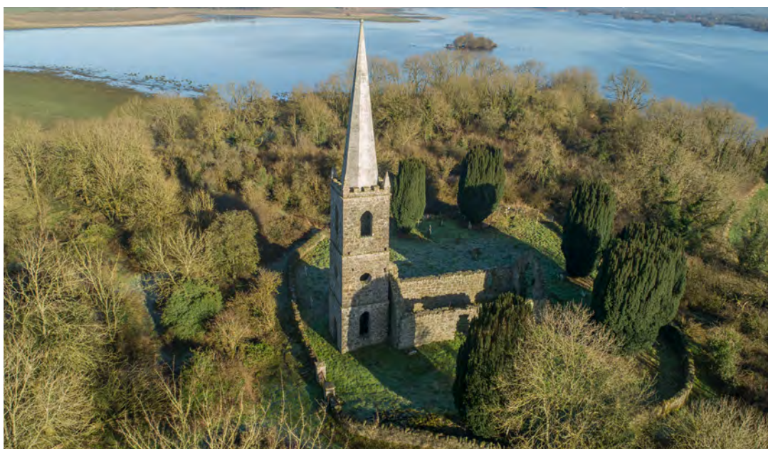
Works at Church Island, Lough Beg (LDY 042:014)
